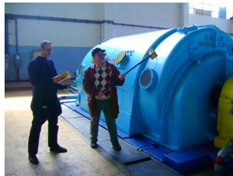
Fig. 6. Test measurement of low-frequency fields emitted by power generation installations.
